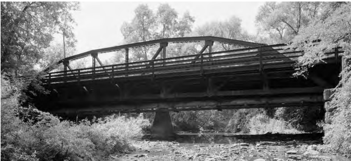
21. Main Street Bridge over Yellow Creek, Poland, OH
