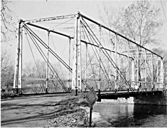
5. Hamden Bridge over Raritan River, Hunterdon County, NJ
