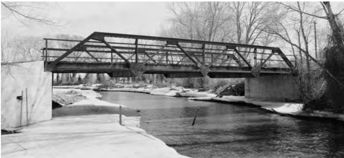
23. Shell Creek Bridge, County Road 57, Big Horn County, WY
