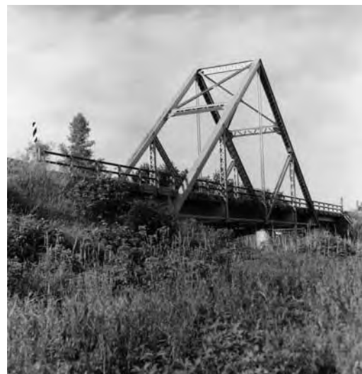
4. Railroad Bridge over Lin Branch Creek, Clinton County, MO
