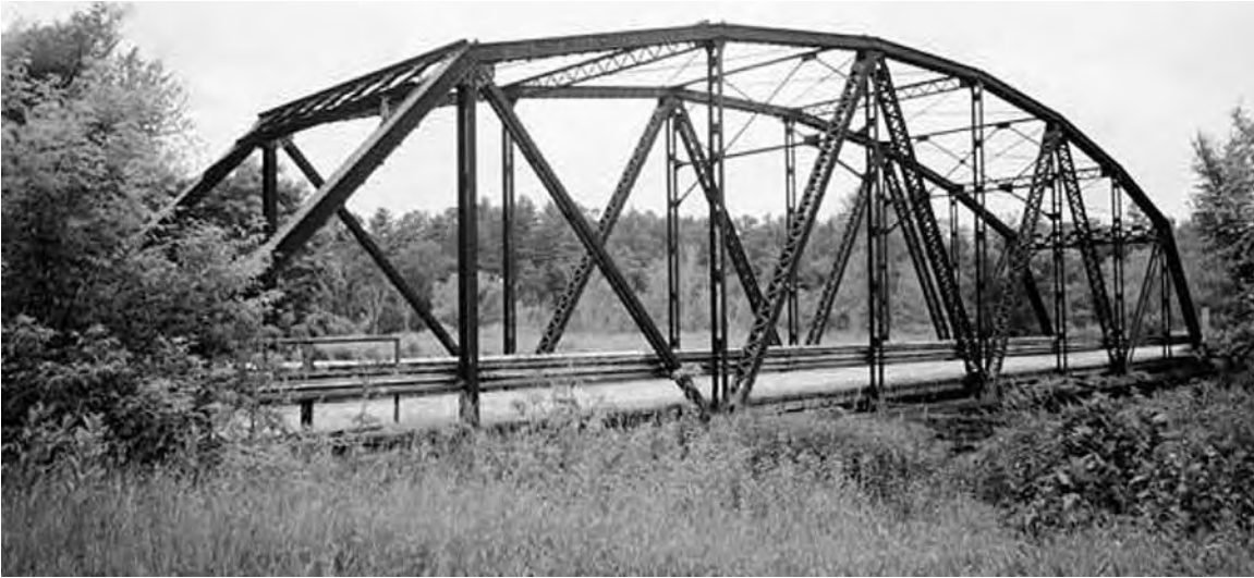
1. State Highway Bridge No. 16 over the Kickapoo River, Vernon County, WI
