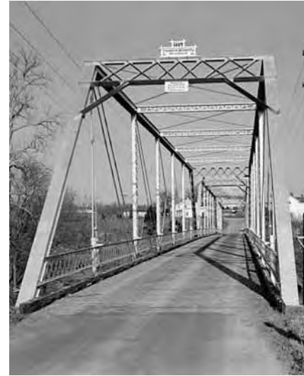
6. State Rt. 256 Bridge over Middle River, Augusta County, VA
