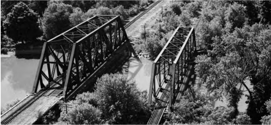
16. Baltimore & Ohio Railroad Bridges, Cattaraugus County, NY
