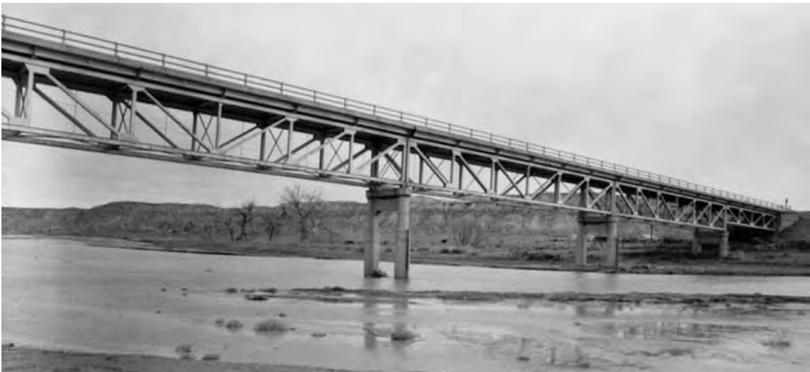
26. Powder River Bridge, Arvada, Sheridan County, WY
