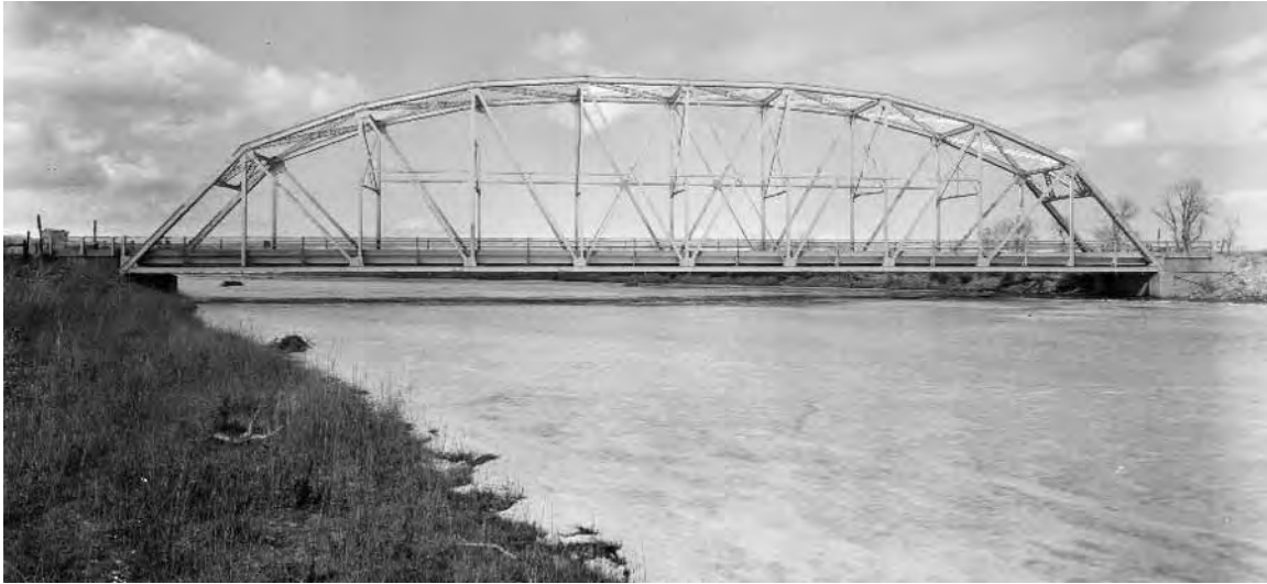
28. Wind River Bridge, Wyoming Highway 132, Fremont County, WY
