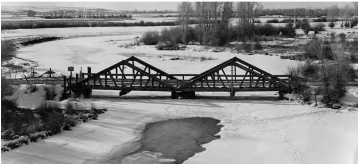
11. New Fork River Bridge, County Rd. 136, Sublette County, WY
