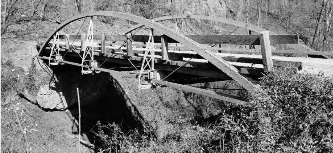
25. Roaring Run Bridge, State Route 657, Bedford County, VA
