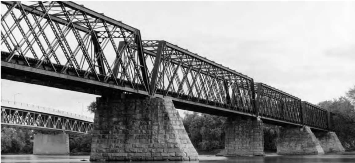
14. Boston & Maine Railroad Bridge, with State Route 9 highway bridge in background, Northampton, MA
