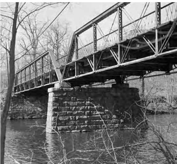
3. Albion Bridge over Blackstone River, Cumberland, RI
